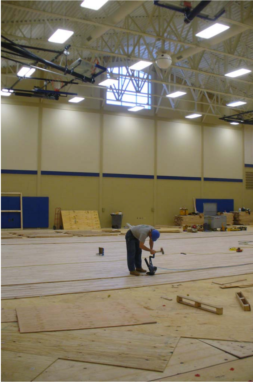
laying gym floor
